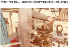
SCREWCUTTING WASHER PLATES FOR A CUSTOMER
