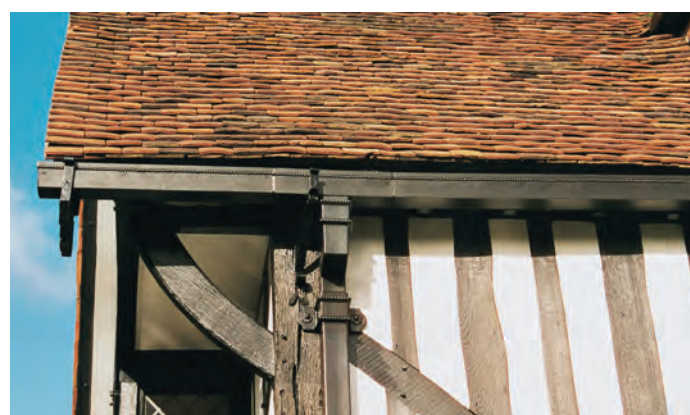
Bespoke GRP gutters were moulded with the rope decoration to be in keeping with the style of this old timber house.
